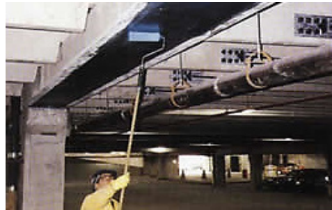
Figure 14. The application of flexural strengthening, [21]
