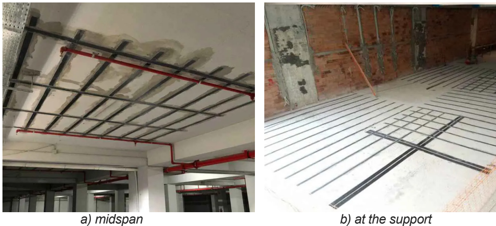
Figure 18. FRP slab strengthening, [14]
