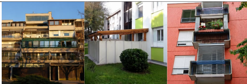
Figure 2. Uncoordinated maintenance works and individual interventions on residential buildings.
